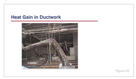
Another source of heat gain in the system may be heat that is transferred to the conditioned air through the walls of the supply and return ductwork. For example, if the supply ductwork is routed through an unconditioned space, such as a ceiling plenum or an attic, heat can be transferred from the air surrounding the duct to the supply air.
