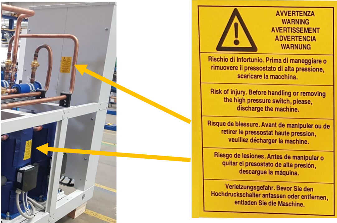
Figure 1 – Indicative position of the signs warning about the necessity of replacing the high pressure switches with the unit void of refrigerant related to the lack of high pressure safety valves
