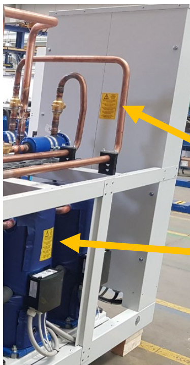
Figure 1 – Indicative position of the signs warning about the necessity of replacing the high pressure switches with the unit void of refrigerant related to the lack of high pressure safety valves
